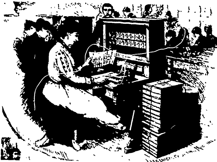
Tabulating the 1890 census by machine. From Scientific American 63 (1890), p. 127.
